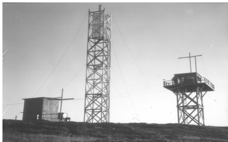
Radio antenna (left) and lookout tower, 1942.
