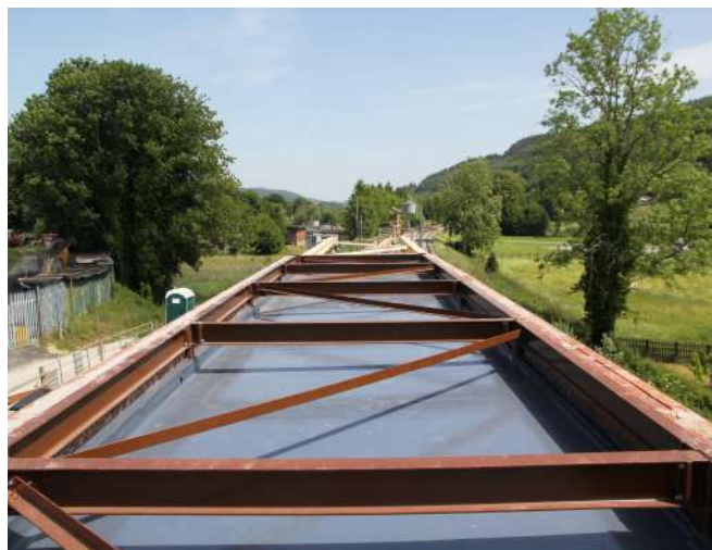
Inner roof, complete with waterproof membrane Photo : PN
