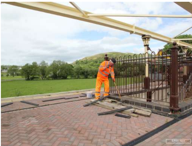
Volunteer, Brian Cope, clearing silt from the platform drains Photo : PN
