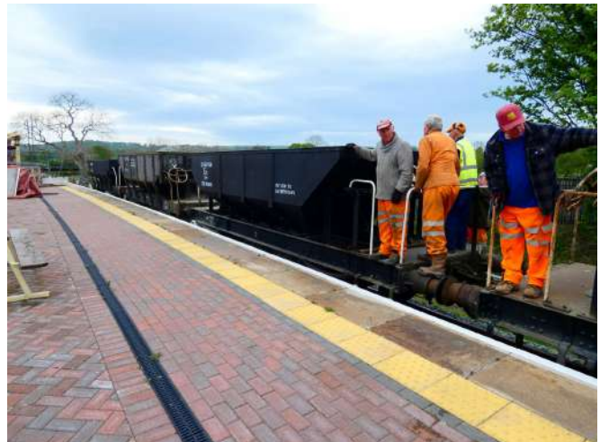
Ballast train in Platform 1 ready for the stone drop Photo : DT
