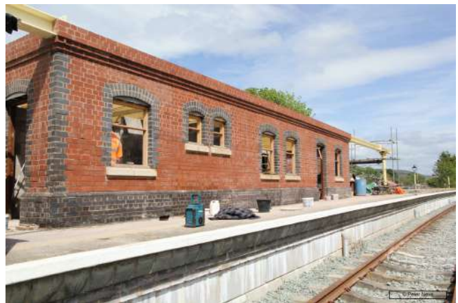
South facing wall, cleaned and scaffold free - very smart Photo : PN
