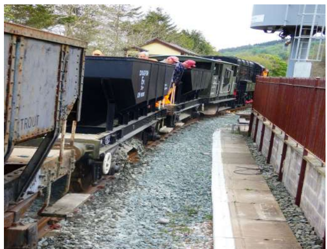
Stone drop underway approaching the east end points Photo : DT
