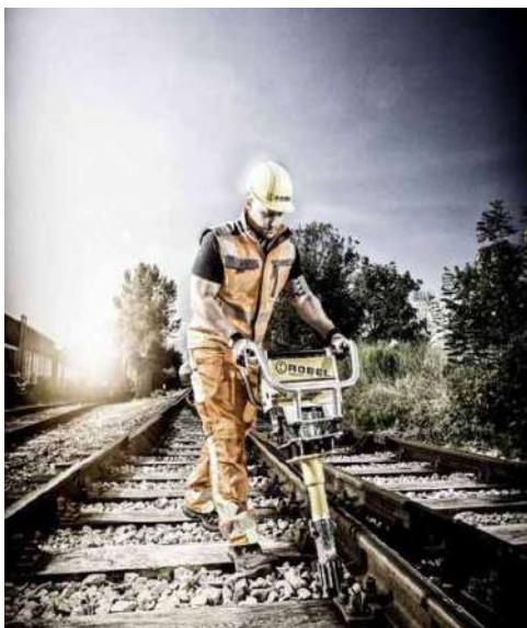
Robel Tamper at work Photo : Torrent Trackside
