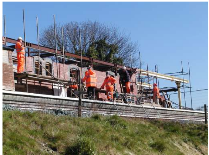
Scaffold along the south wall
