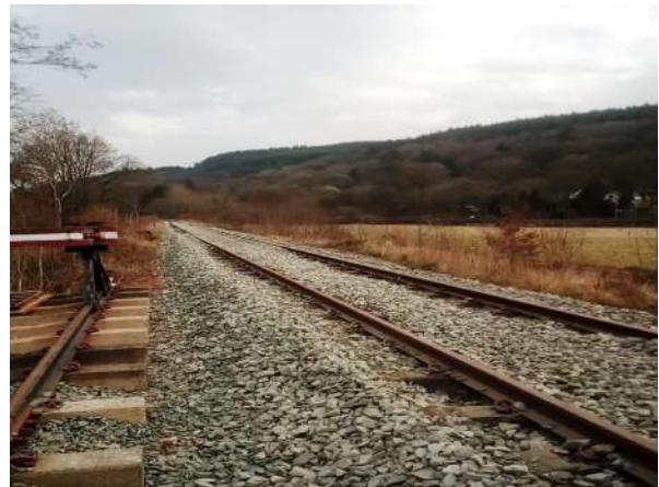
Ballast to the east of the station after the drop Photo : PR
