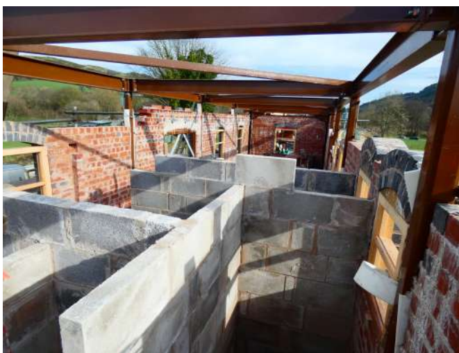
Internal walls for the toilet/washroom facilities take shape Photo: DT
