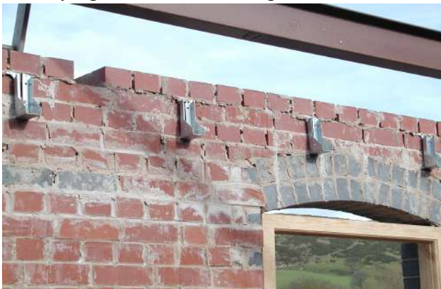
Roof truss hangers in position Photo: PR
