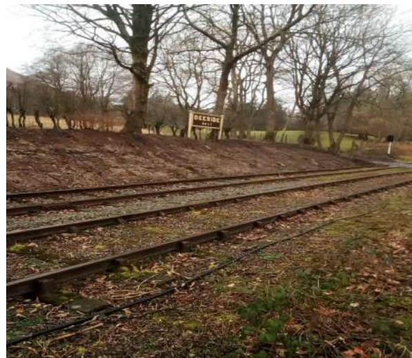
Platform now removed and the cutting graded back ready for sowing
