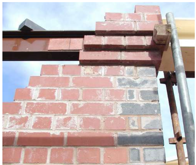
Brickwork stepped out to enclose steel frame Photo : PR
