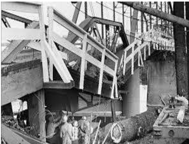
Damage from the Columbus Day Storm ( Freda )
