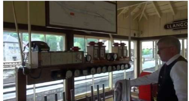
Block shelf in Llangollen Station Signal Box
