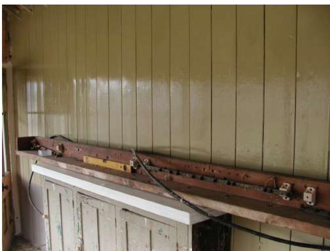
ICupboard restored and painted with block shelf resting on top with power cable Photo : PR
