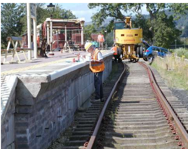
Wayne adds white lines to edging slabs on platform 2 Photo : PR
