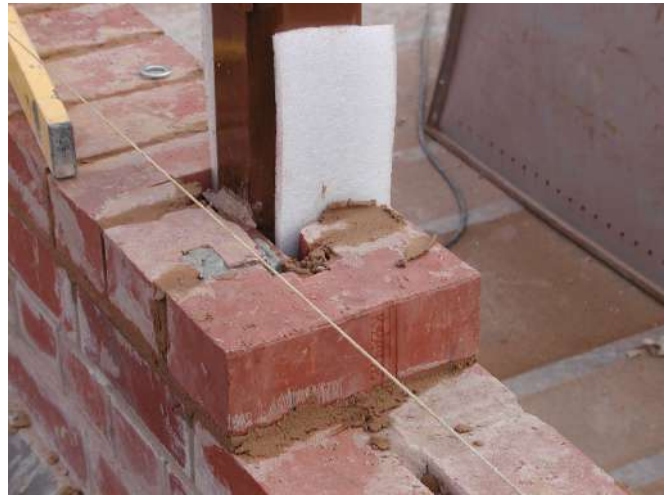
Slotted bonding of the brickwork . Bonding resin shown in the middle of the picture Photo : PR
