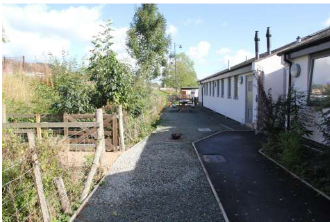
Relayed pathway behind the Health Centre after regrading the pipework Photo : PN
