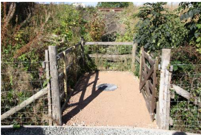
New receiving chamber - centre of picture Photo : PN
