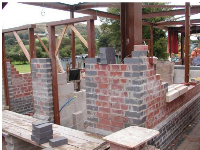
Internal walls taking shape in the station waiting room Photo : PR
