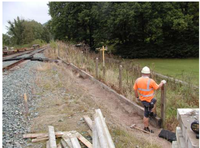
Bomac ramp walk now removed. Crossing Bomacs visible top left
