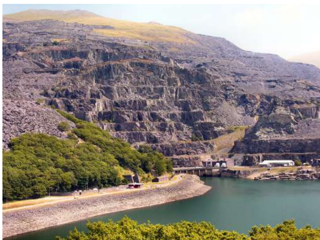
Part of the power station as seen on the exterior of Elidir Fawr. Photo : Dennis Egan
