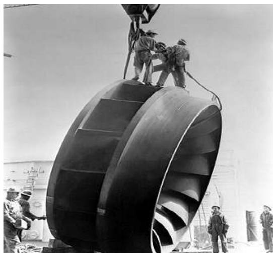
Francis turbine runner- the bit that generates the power
