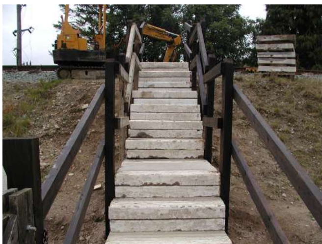
The East End steps now with posts and rails added Photo: PR
