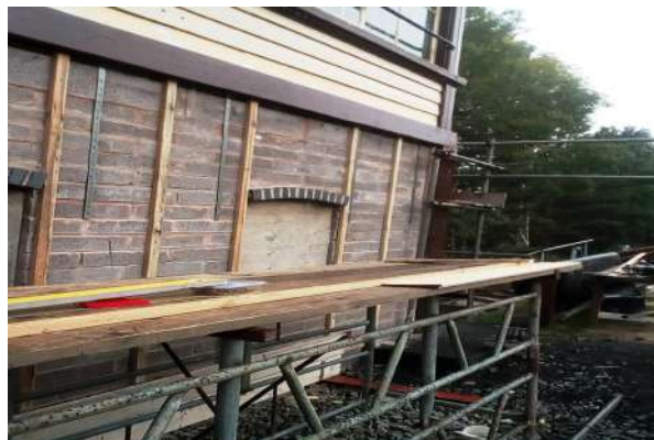
Cladding support battens in place
