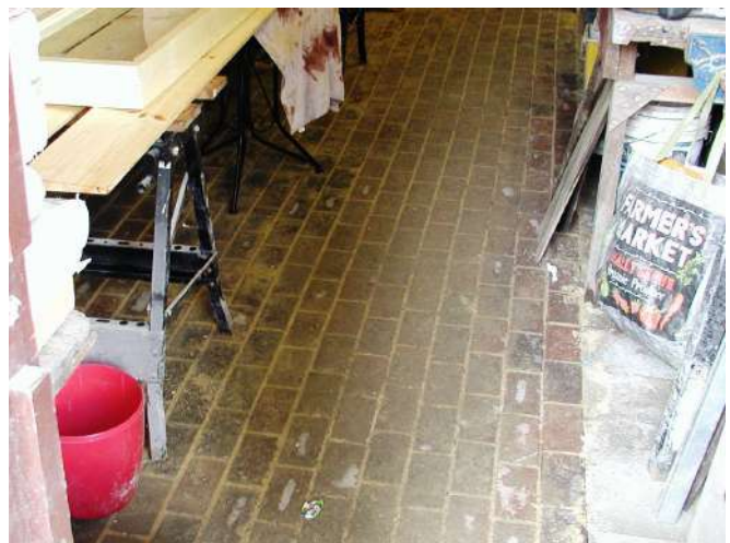
New block floor for the signal box basement
