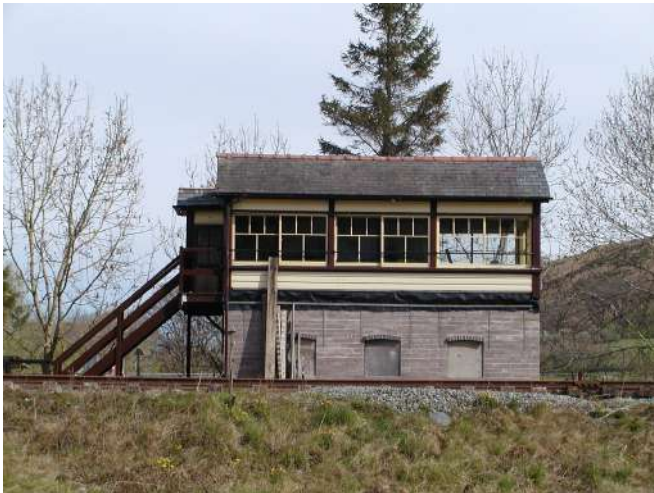
Signal box awaits external cladding
