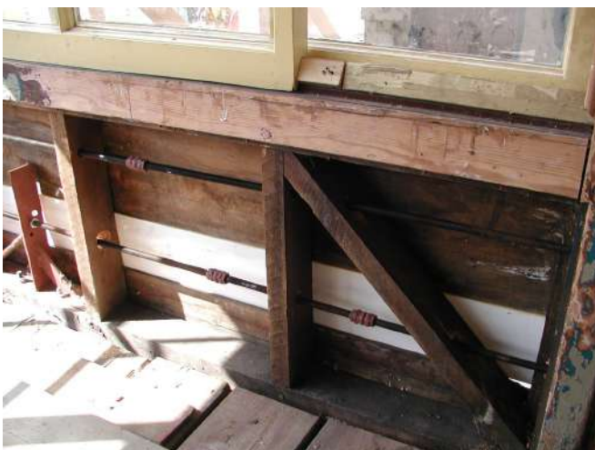
Steel frame and tie bars to bind in the corner posts
