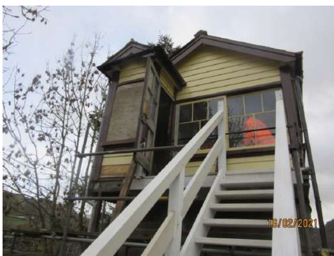
SB Stairs with hand rail and porch door open Photo: PM
