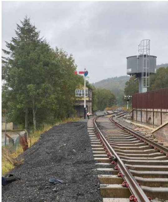
CN 24 & 11 UP starter Platform 2 and Shunt signal to Up siding Source : HJP
