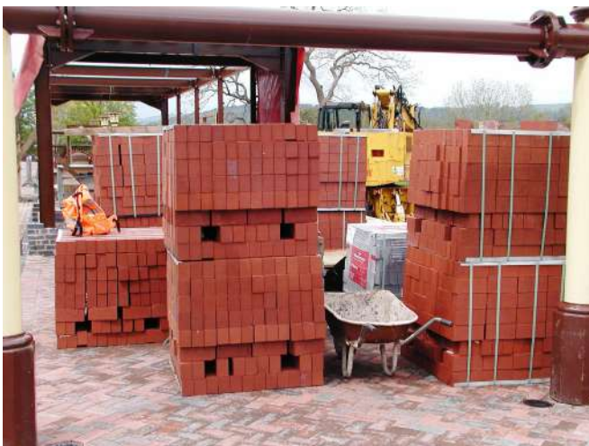
Standard red bricks awaiting their turn Photo : PR
