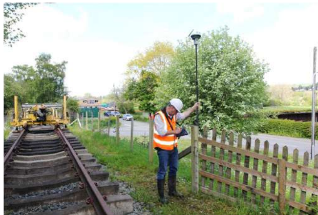
Ian Hayward, holding GPS receiver and key pad makes a start on the mapping of Corwen's new station Photo : PN
