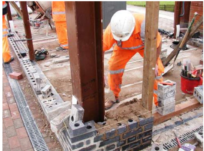
Peter Jump building up around a corner post Photo : PR
