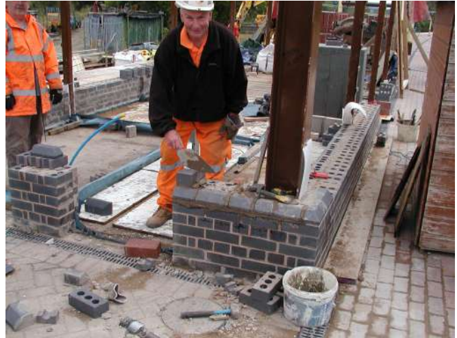
Peter Jump fitting the plinth bricks at another corner post
