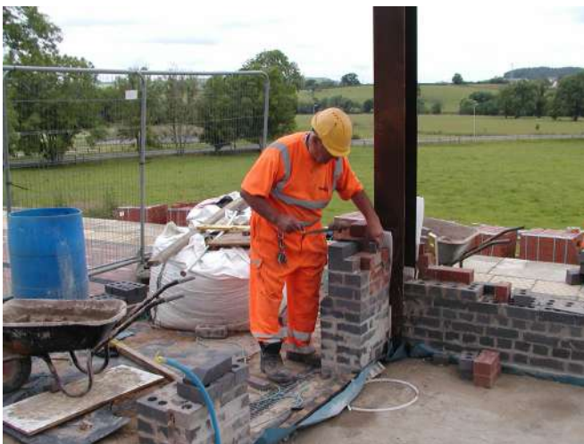
John Mason building up a corner post
