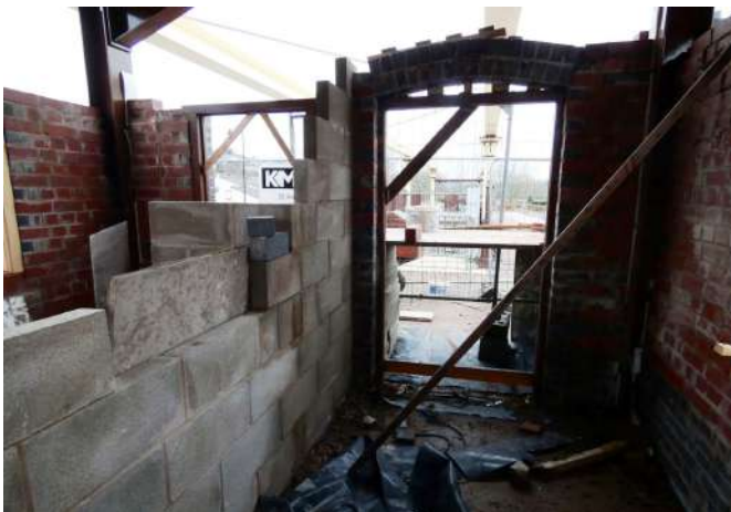
West end of building - internal wall Photo: DT
