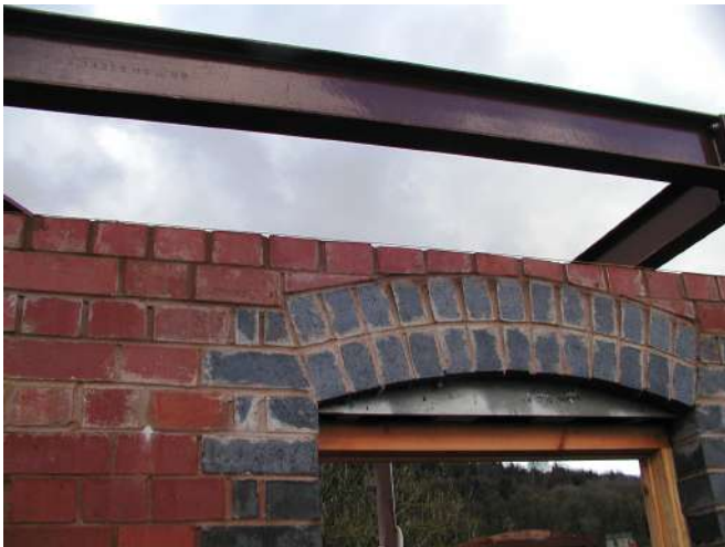
Thin brick course across the top of the window arch
