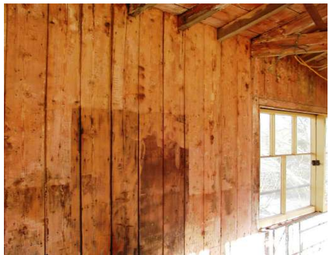
With old paint removed original wood still in excellent condition
