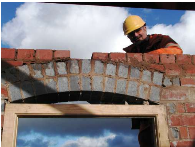
Ready for the last brick over the arch
