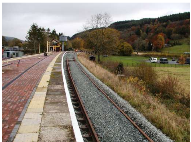
Ballast complete in the down platform - looking east Photo : PR
