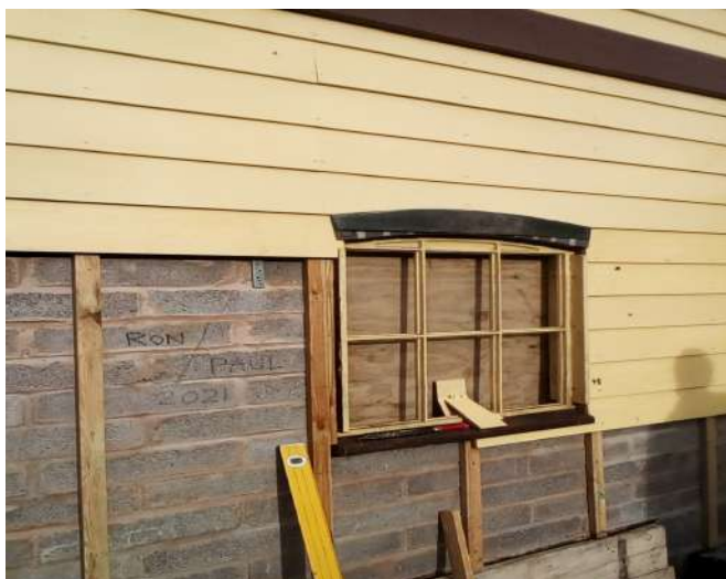
Signal Box cladding neatly surrounds locking room window Photo : PR
