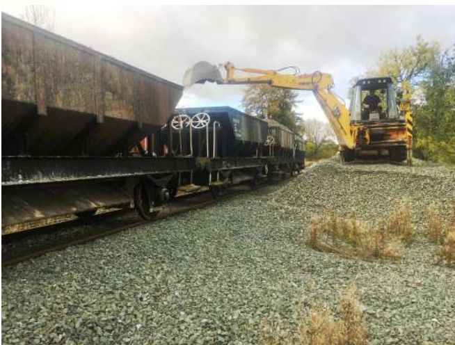
"Two down Two to go" - Loading Ballast at Bonwm Farm Photo : PR
