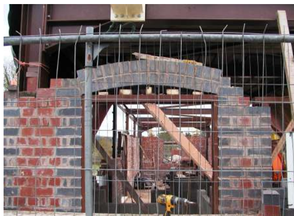
Archway takes shapes over the west facing doorway Photo : PR
