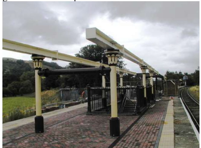
Carrier beams in place bolted to the building frame
