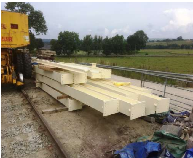
Carrier beams ready for installation Photo: RDG
