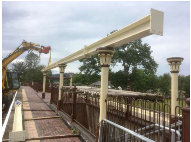
RRV gets to work putting the carrier beams in place
