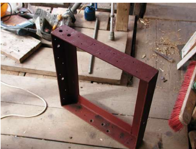
Steel frame to support the woodwork (see photos above – page 2) Photo : PR
