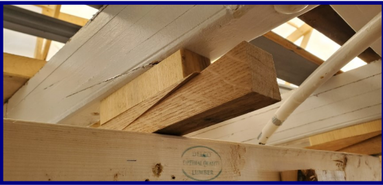
Beams have been shimmed to eliminate sagging. This technique gained approximately 3/4" of height.
