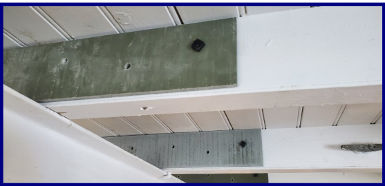
Plates are added to reinforce the joint where the replacement beam joins the old beam. These will be painted white.
