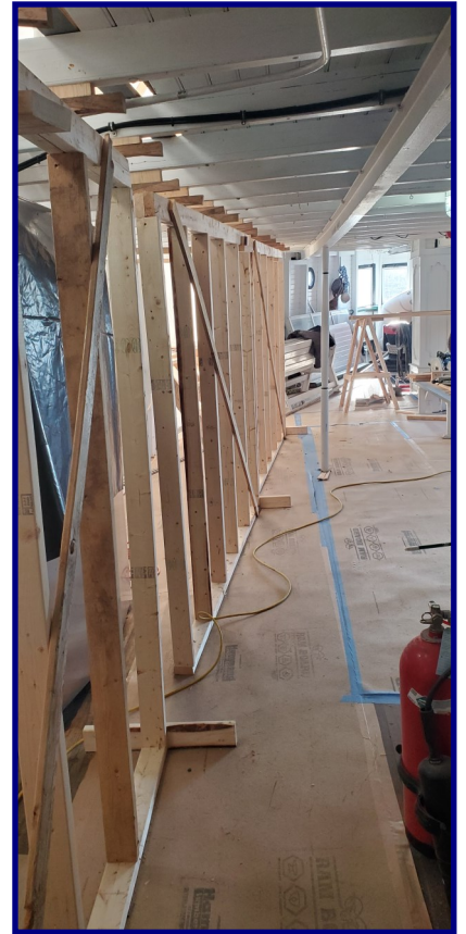
Supports line the port side of the cabin to raise sagging beams (see photo, upper left corner of page).
