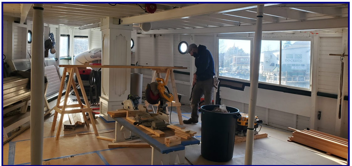
A carpenter from The Shipyard in Boothbay Harbor saws lumber in preparation for "laminating" beams. In this process, several layers of lumber are stacked and glued together, increasing the strength of the beam.
