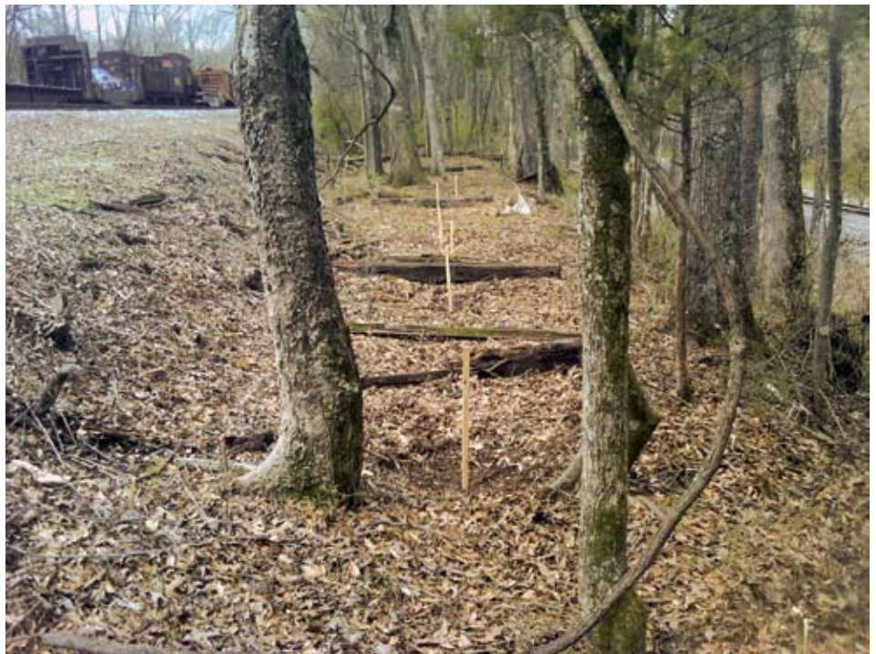
The roadbed of the Dalton Junction connection as it appeared in early 2013, looking west. The stakes indicate the location of some timber pilings. The TVRM-ET&G main line is at left; cars are stored on the siding at McCarty. The track at right is CSX Tyner Branch, constructed by NC&StL to serve Volunteer Army Ammunition Plant at Tyner during World War II. MARK BRAINARD PHOTO
