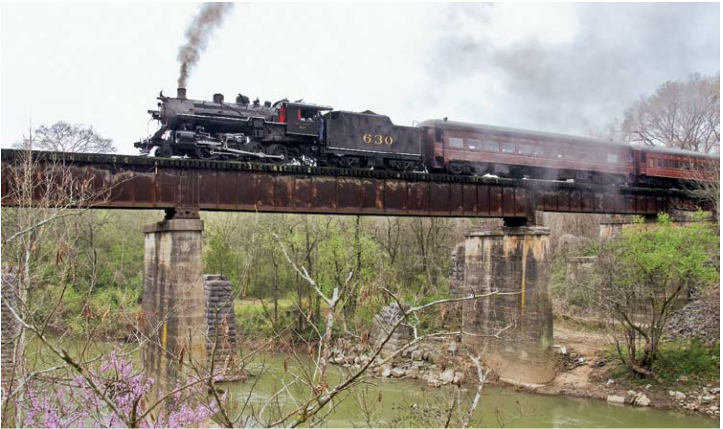
Southern/TVRM 630 crosses South Chickamauga Creek eastbound in spring 2012. Visible beyond the concrete piers supporting 630 and her train are stone piers from an earlier ETV&G bridge that was removed when the Southern modernized and relocated the right-of-way around 1912. The stone pier partially obscured in the center of the picture is believed to rest on the westernmost foundation of the original ET&G stone arch bridge that existed during the Civil War. CASEY THOMASON PHOTO
