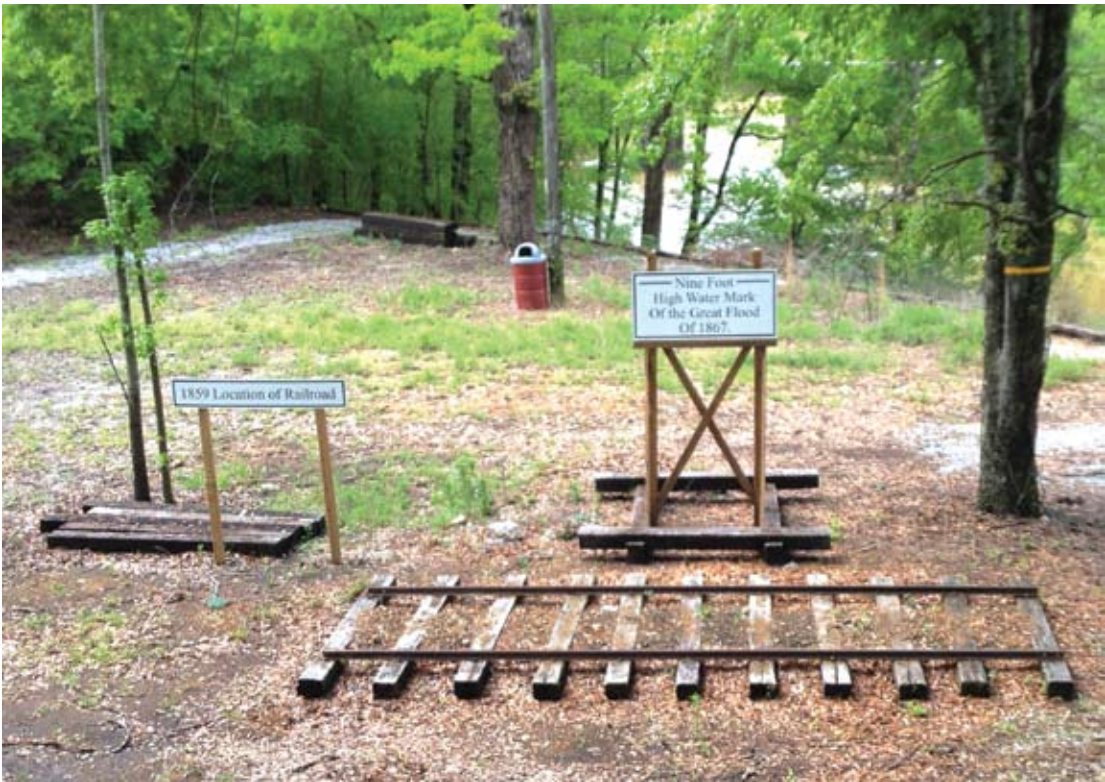
The reconstruction of a short segment of Civil War-era track on original roadbed of East Tennessee & Georgia Railroad is just one of many historical presentations found at TVRM. This one is on the east bank of South Chickamauga Creek (visible in background). Laid to 5-foot gauge, the rail is appropriate for the Civil War era and is spiked directly to untreated cross-ties. Behind the trees to the left is a small bluff overlooking the location of the ET&G bridge and Dalton Junction. This view from the TVRM main line was taken in March 2013. BILL SCHAFFER PHOTO
