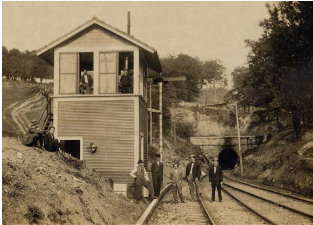
Southern Railway's VM Tower is seen in this 1915 view several hundred feet west of Missionary Ridge Tunnel. In 1912, Southern straightened and double-tracked its main line between Chattanooga and Ooltewah except through the tunnel. VM Tower was manned by round-the-clock operators, who controlled train movements over the two main line tracks that converged at each end of the tunnel. The home signal for northbound trains, for example, was an upper-quadrant semaphore behind the photographer's right shoulder. When the signal was in the "stop" position, a switch point derail opened to divert to the ditch any trains that did not heed the signal. The lower-quadrant semaphores at the tower indicated whether or not a passing train needed to pick up train orders. The three men in the middle of the row all worked as operators at VM Tower: from left to right, Ira K. Hall, Calvin Cash, and Fred Redwine (who later became a local attorney). Some time later, possibly in the 1930s, control over movements through the tunnel was transferred to Citico Tower near downtown Chattanooga, and VM Tower was closed. TVRM collection.
